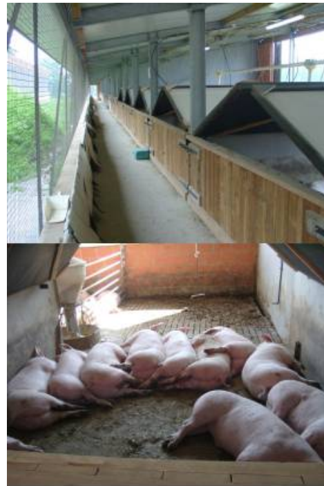
Figure 3. Example of an open front unit with free ventilation and insulated sleeping boxes.
